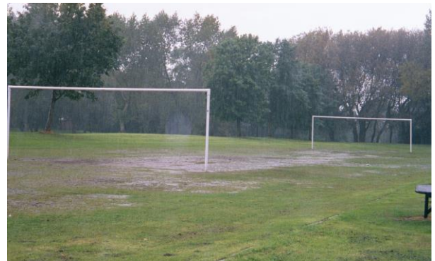
Many parks were built on poor quality land. Poor drainage remains a problem, here on the football pitch at Philips Park
